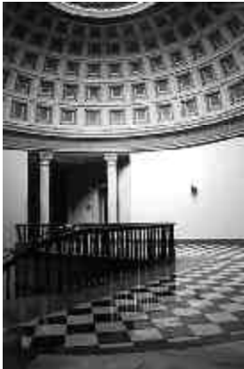
OEOB skylit stairwell
